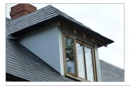
White 9016 3mm Alupanel has been used as the Dormer cheeks on this building. It acts as an impressive weather shield and also provides an element of sound proofing and insulation. The panel has been cut to size and routed, all on-site, then simply fixed to the Dormer construction.
